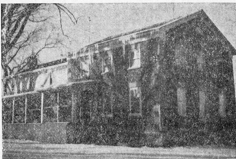
State School farm house on the Vienna St. Rd. was built with medium field stones of all colors and a cobblestone foundation.
